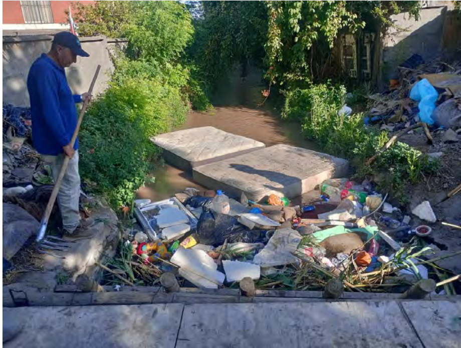
Figure A.IV: Irrigation Infrastructure Maintenance
